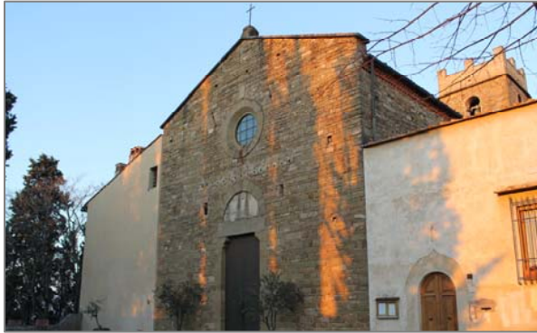
The facade of S. Margherita a Montici
