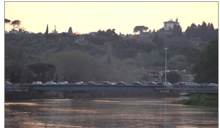
S. Niccolò Bridge with Belvedere Fort in the background
