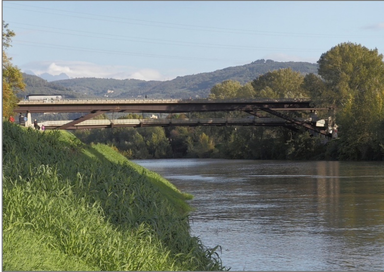
The Varlungo Bridge
