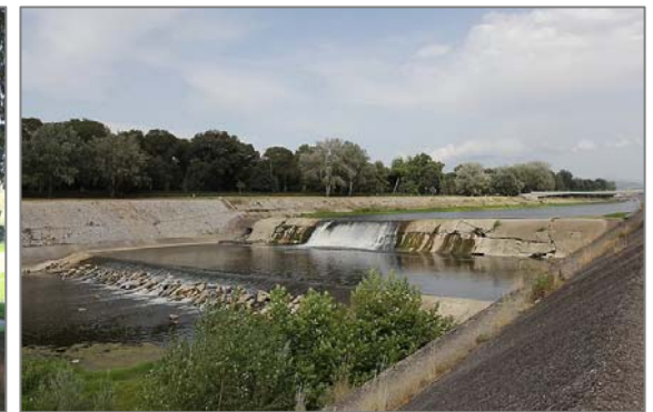
The Isolotto weir
