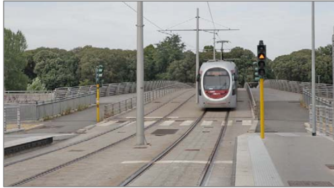
The bridge of tram line 1
