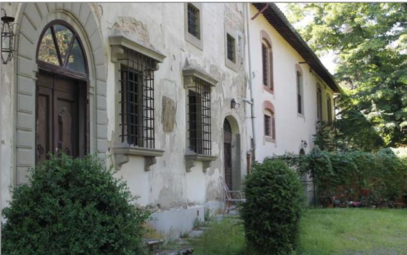
Villa Lisi: partial view of the facade
